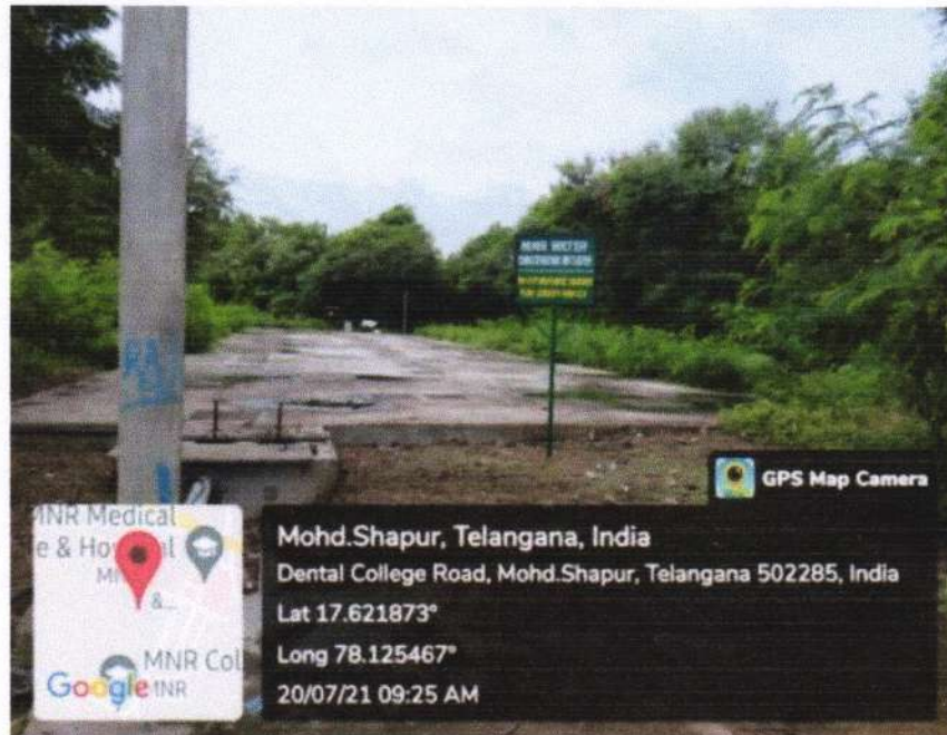
RAIN WATER HARVESTING
